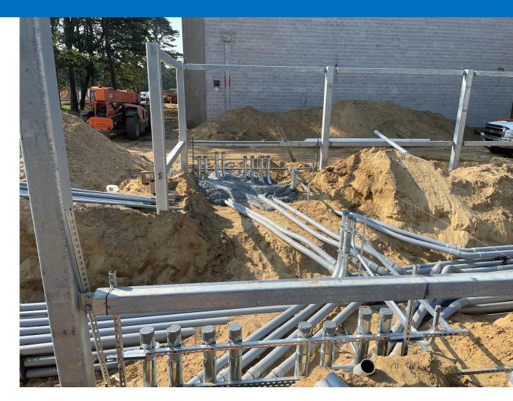
E building back filling and compacting UG plumbing and electrical
