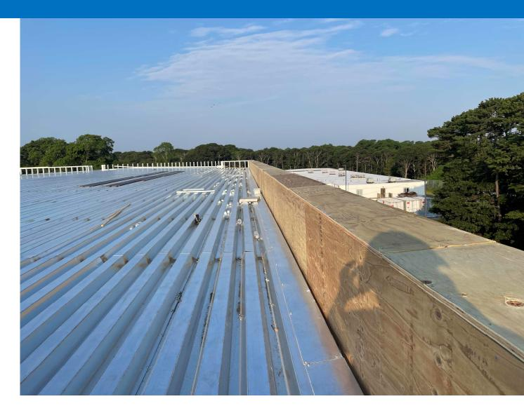
E Building exterior installing FCEC clips for Metal studs
