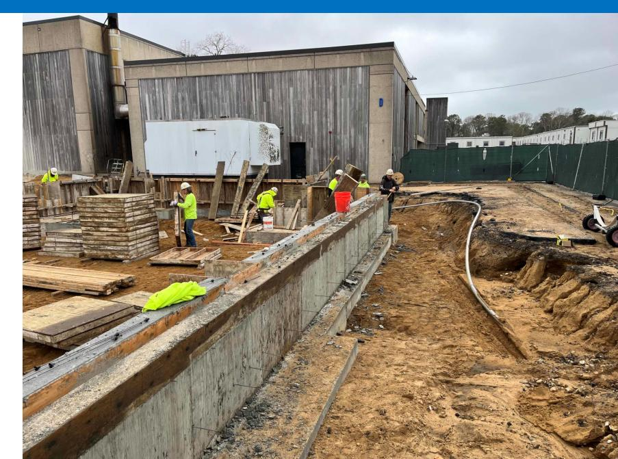
E Building foundation wall concrete placement
