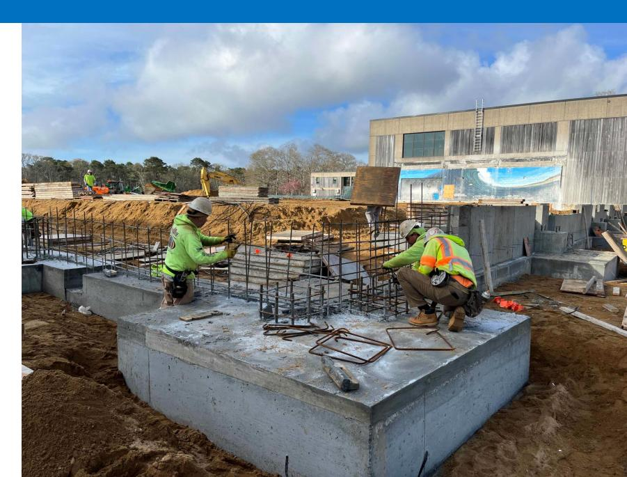
F Building line excavation to bottom of footing elevation
