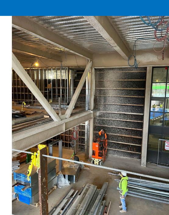
E Building south wall elevation precast wall panel installations.
