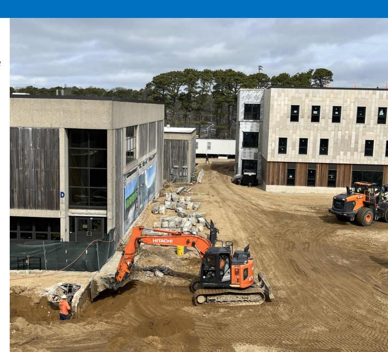
Backfilling at stripped sidewalks in the courtyard.
