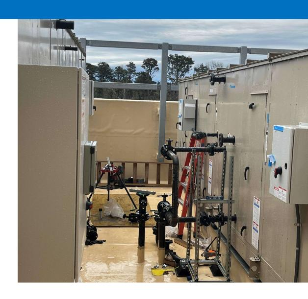
Welding pipes on stands and in place mechanical room 1st floor E-Building.
