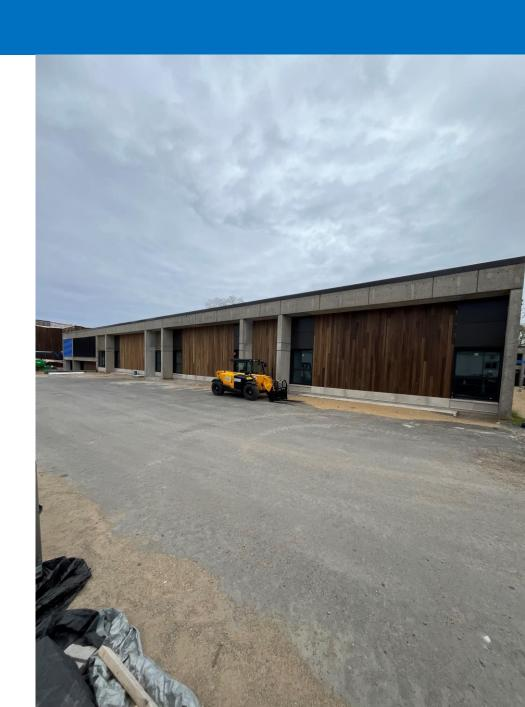
D building North elevation Cambia vertical siding installation completed
